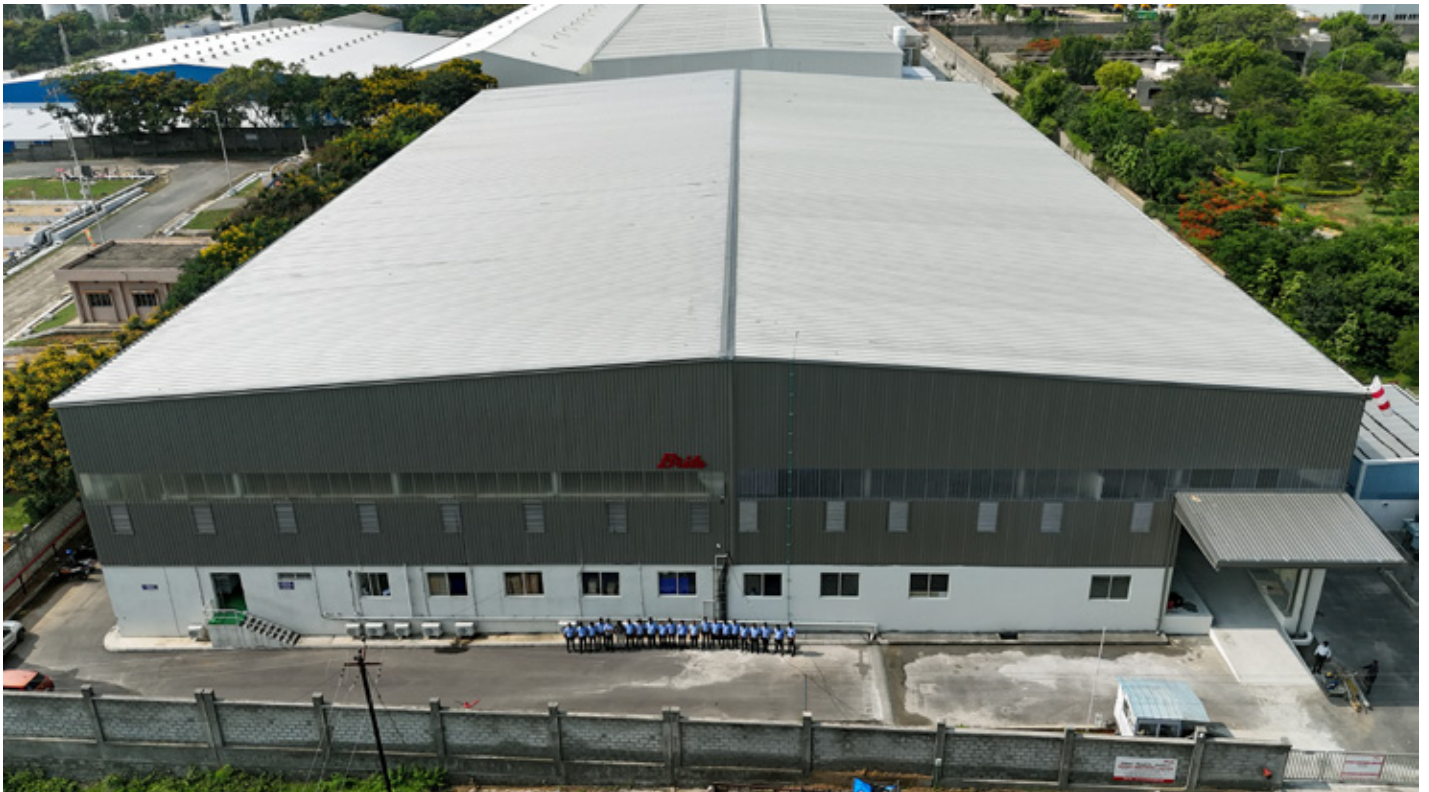
Extended manufacturing facility at Hosur in 2025
